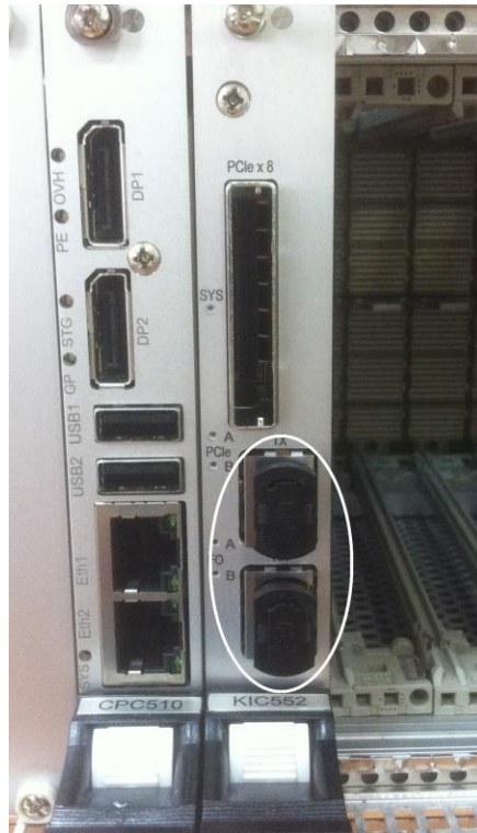
Fig. 3-6: Connectors for optical cables with the installed stopping plugs
