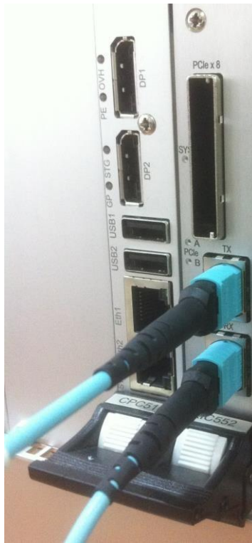
Fig. 3-8: Connection of QSFP optical cables
